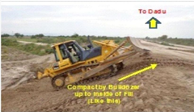
Slope Compaction by Bulldozer (21 ton)
