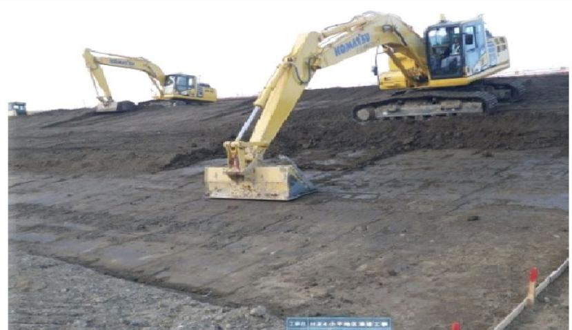
Slope Compaction by Hydraulic Excavator (Long-Arm)
