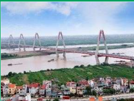
Viet Nam - Nhat Tan Bridge Type: 6 span continuous cable-stayed bridge
