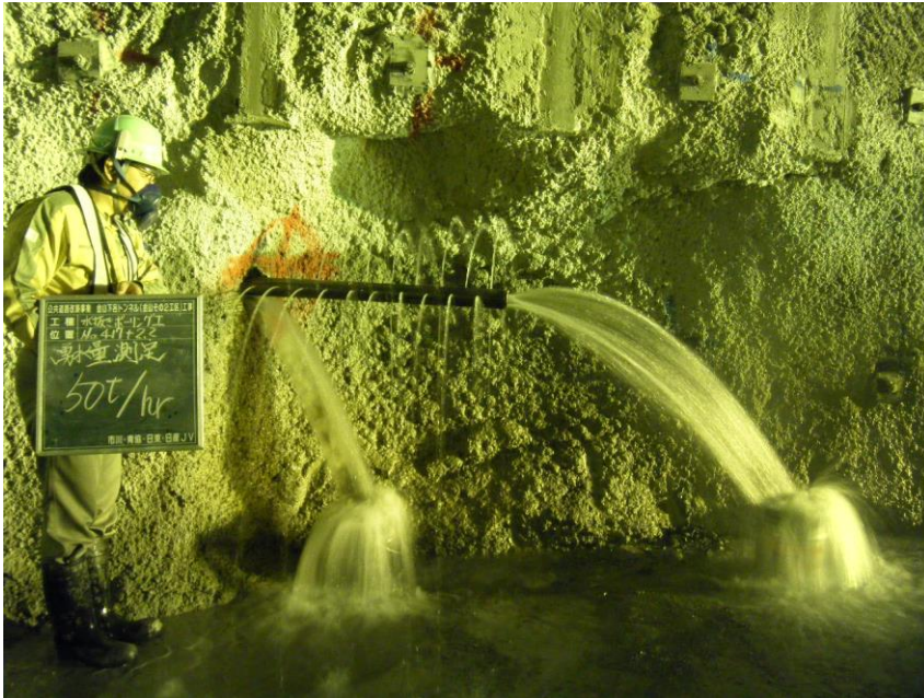
Drainage boring of Kanayama Gero Tunnel
